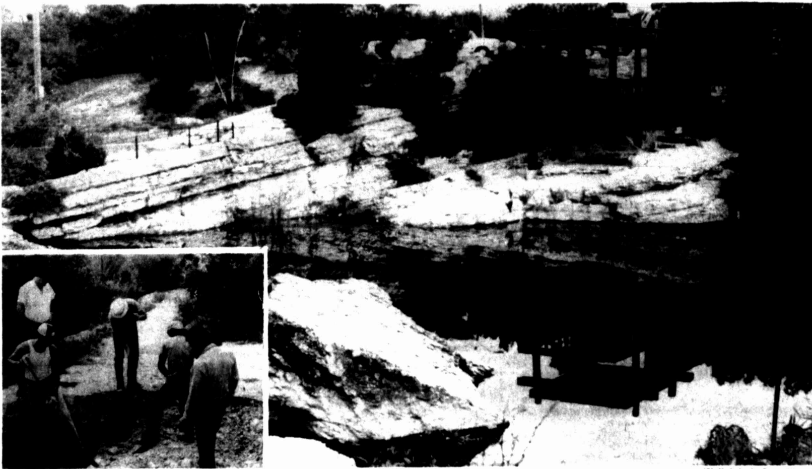
SPRING CLEANING — The site of the historical spring from which Big Spring derives its name is being drained and cleaned. City Manager Don Davis explains that two pumps that bring nearby well water into the spring had broken down and since they were down "we felt like this was a good opportunity to drain it (the spring) and give it a real good cleaning." The old
