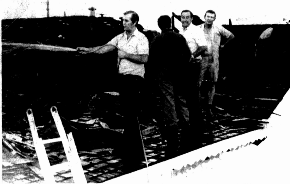
HEAVY DAMAGE — The Jackie Rinard home, Route 3, Box 86, was heavily damaged in a fire at 5:38 p.m. Friday. Here, Truman Mason sprays water on the roof of the home, which sustained the heaviest damage. Neighbors
