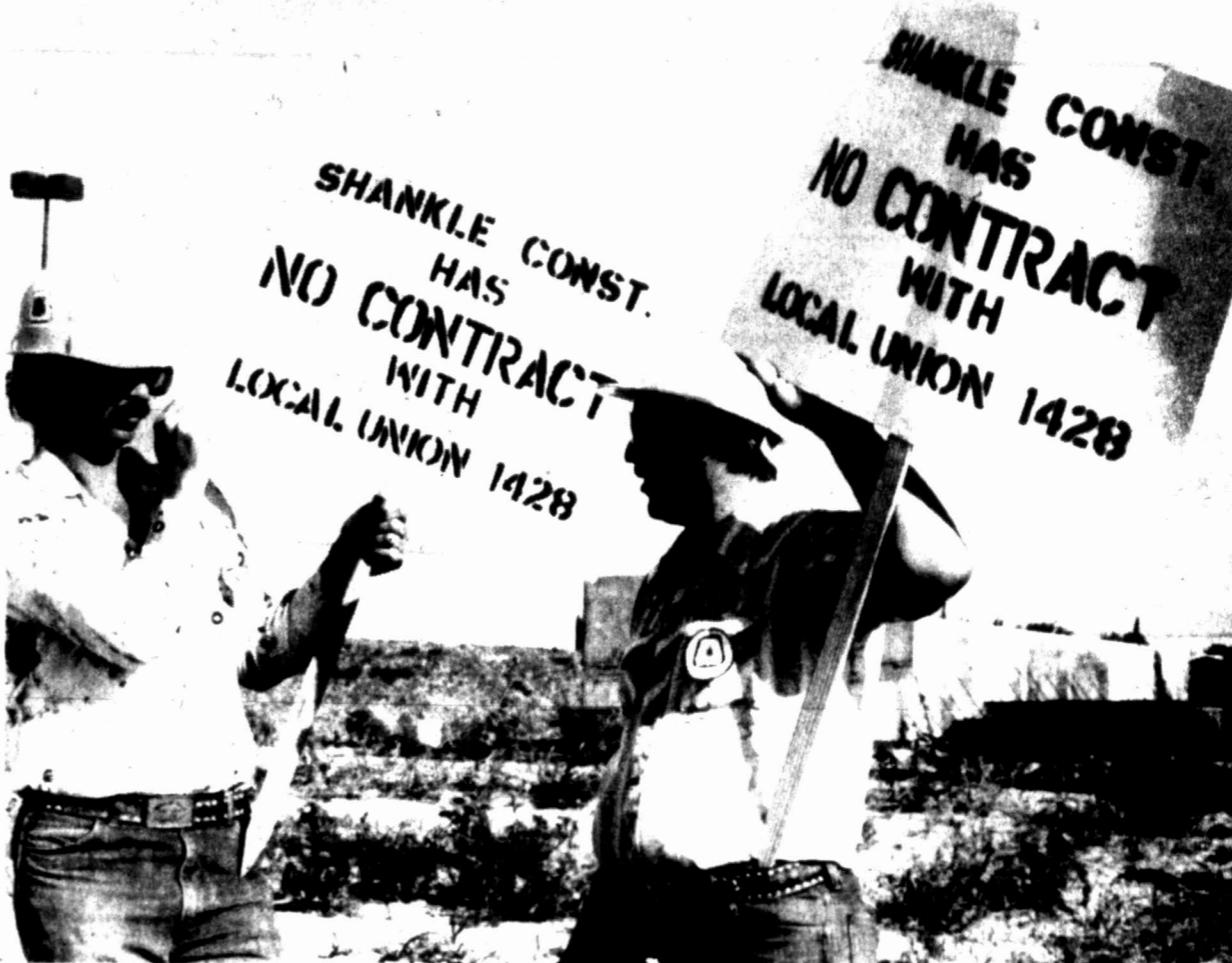
CARPENTERS' STRIKE — Terry Purcell, left, and his brother Jim manned the picket line at the mall construction site on east F.M. 700 this morning. Striking carpenters are asking for a two-year pact giving them a
