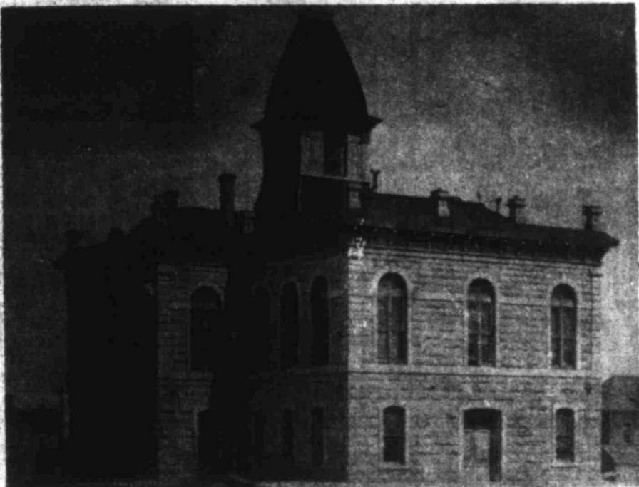
settled their debt for half that amount. The second courthouse (lower right) was constructed in 1908, after the original stone structure had been declared inadequate and unsafe. This one was constructed of red (Pecos) sandstone, a material popular at the time.
