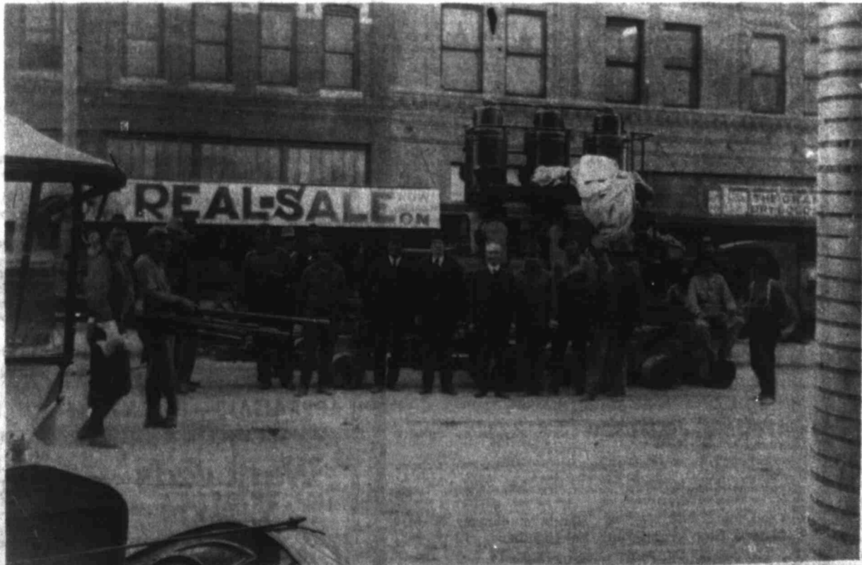
FIRST WATER PUMP — The first city water pump ever installed in Big Spring is shown on a dray with wooden wheels following its arrival here in the early part of the 20th Century. Copious water was to flow shortly later from wells in what is now Comanche Trail Park. Rome wasn't built in a day and getting this pump in place and "on stream" took a long time, too. Lawrence Bell supplied this picture.
