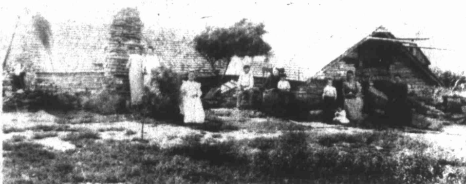
VINTAGE HOUSING COMING BACK INTO VOGUE — One of the more popular type of housing built in this area in the late 1900s was the dugout, built partly into the ground as protection against the savage winds and the numbing cold that could hit the area from time to time. It was much easier to heat than conventional housing and proved cooler during the summer months. Now, with energy costs continuing to escalate, the dugout-type of structure is again becoming popular with Americans.
