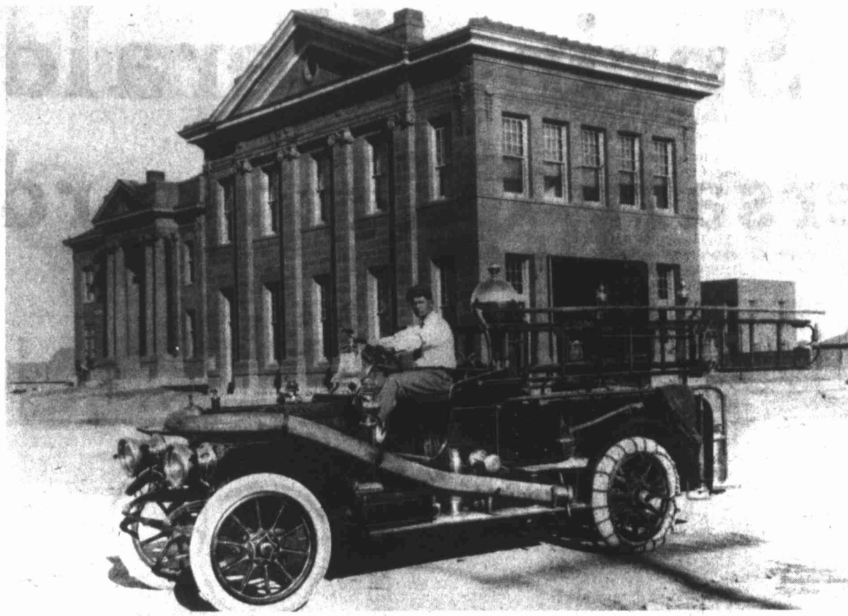
PRIDE OF THE WEST — In 1907, Big Spring had a disastrous fire, and the newly-founded city government resolved to do something about fire protection. It bought the Thomas Flyer pictured here — advertised as a "fire engine, hose wagon and chemical truck — self propelled." It became the first motorized, mobile piece of fire equipment in the state. Here, the late G. Wyatt
