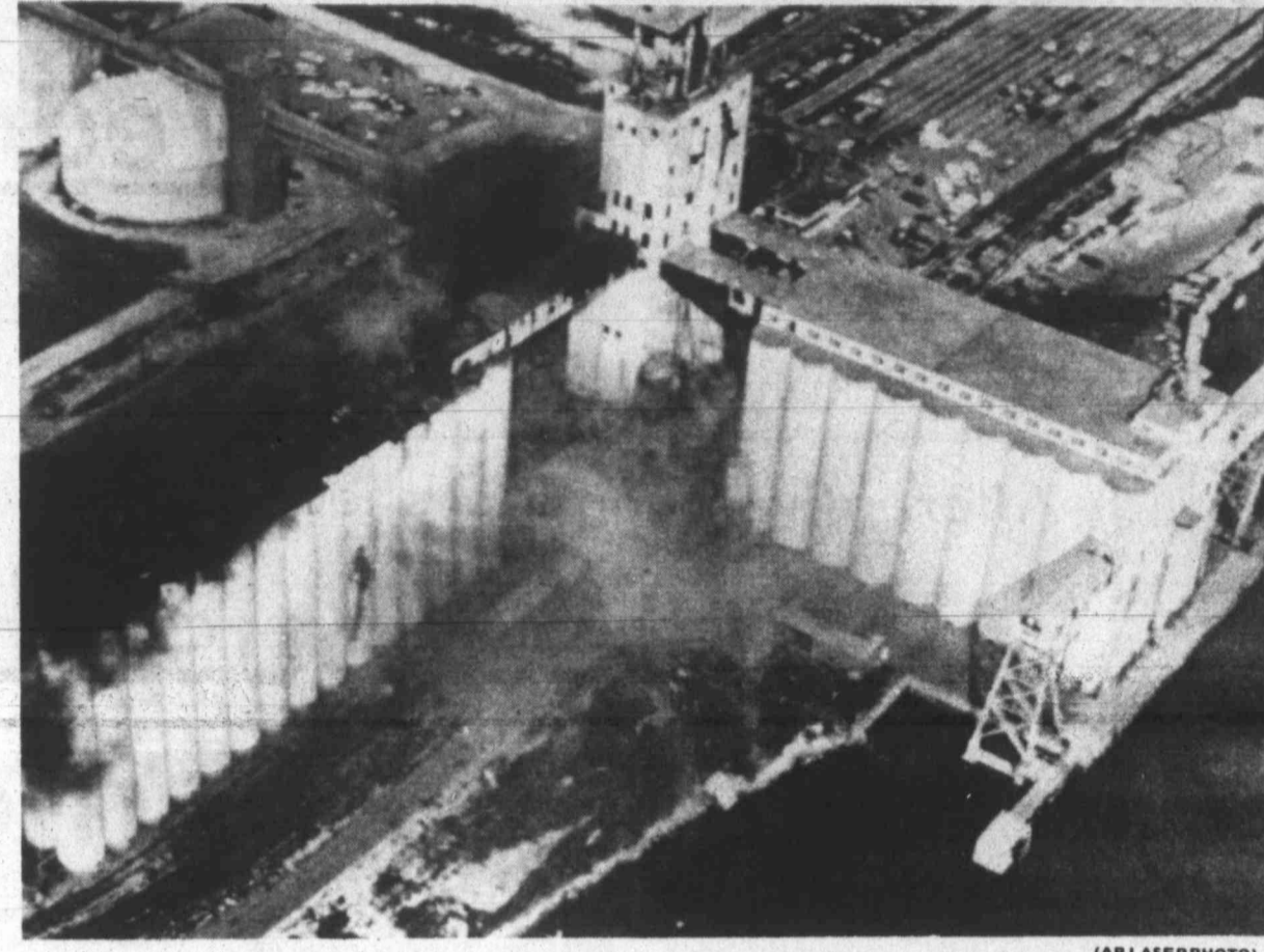
GRAIN EXPLOSION — Grain silos continue to burn after an explosion ripped through the Corpus Christi Public Grain Elevator in Corpus Christi, Texas Tuesday afternoon. The explosion and fire killed at least three
