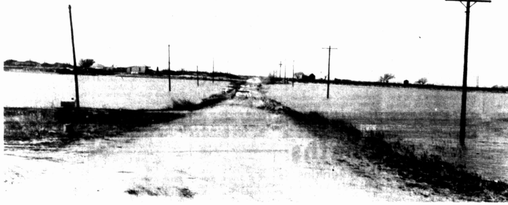
IMPASSABLE ROADS — Several county roads in the Fairview and Knott areas of Howard County became impassable due to heavy rains in September. Pumps were borrowed from the State Highway Department to clear an area
