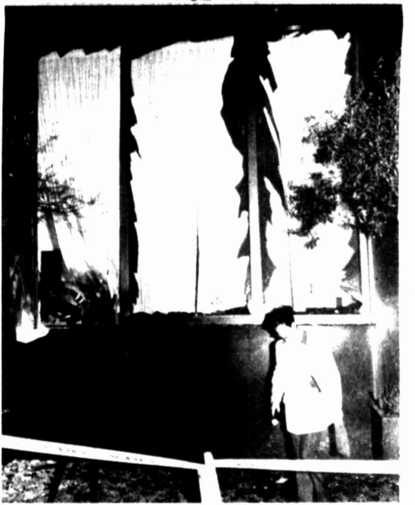
SCENE OF BOMBING — San Francisco squad member looks for clues to the early morning explosion at the Iranian bank in S.F.'s financial district. The Bank Melli suffered minor structural damage. Large plate glass windows of the bank and surrounding buildings were blown out.
