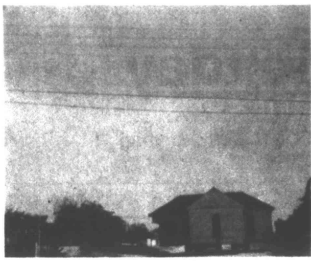
ROLLING HOME — Power lines posed a problem in moving the new day care structure from 15th and Main to Northeast Eighth and Rannels. The only solution was to remove a portion of the roof.
