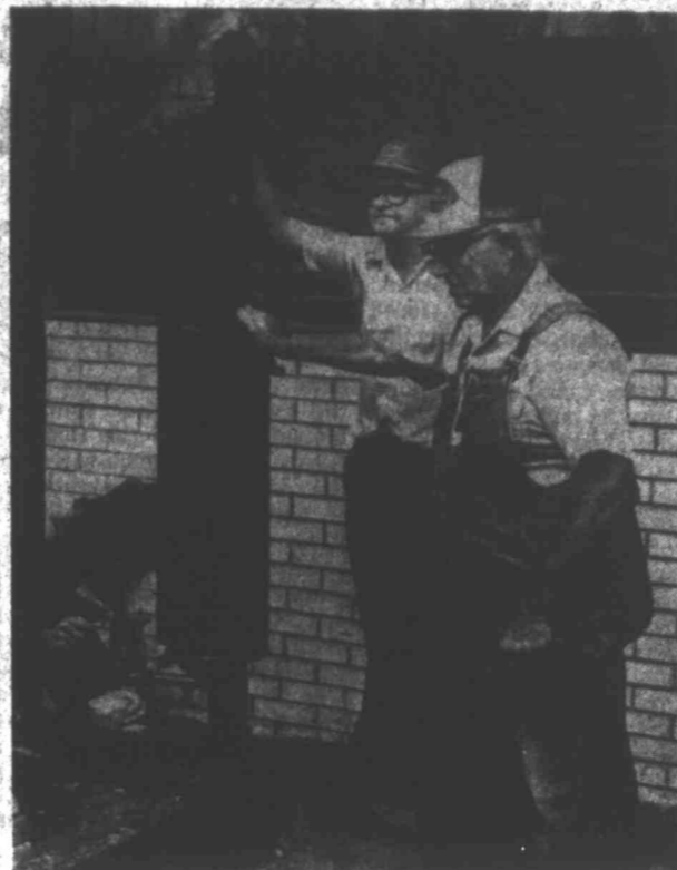
MUSEUM OPENING — B.H. (Blackie) Harris, right, a 45-year veteran of the East Texas oil fields, oversees final equipment installation Wednesday in preparation for the opening of the East Texas Oil Museum on the Kilgore College campus here. The museum, built by Placid Oil, will be dedicated Friday afternoon as part of the 50th anniversary of the discovery of oil in the Daisy Bradford No. 3 well near here which was the start of the East Texas oil boom.
