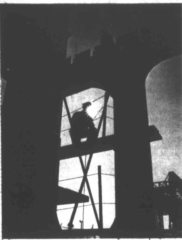
DOWN TO THE SEA — But not yet. An employee of Tenneco Inc.'s Newport News Shipbuilding subsidiary does some preparatory work on a ship in the earlier stages of construction at the Virginia shipyard.
