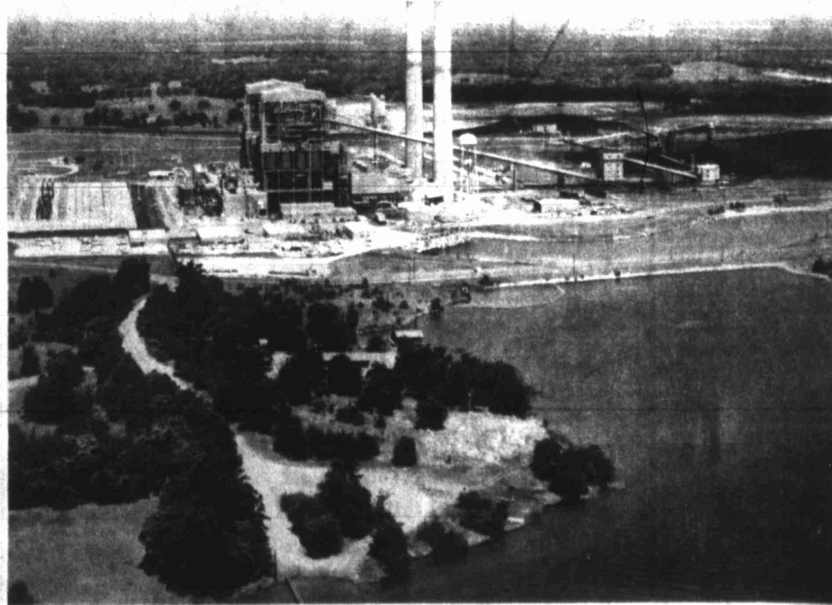
BIG BROWN STEAM ELECTRIC STATION — In Freestone County near Corsicana with its two 575,000-kilowatt generating units, was the Texas Utilities System's first jointly-owned lignite-fueled power plant. It, like the
