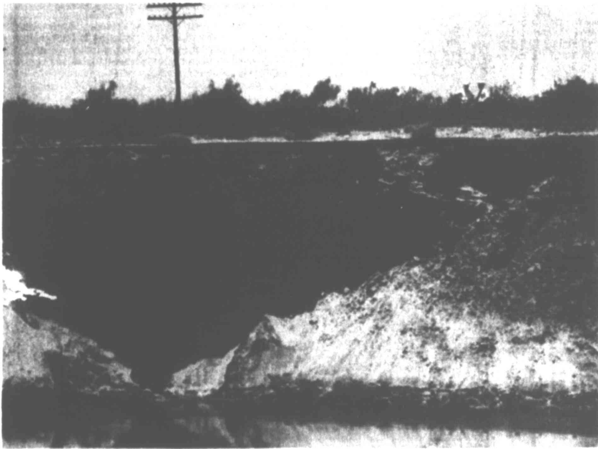
DIRT WALLS CONTINUE TO FALL — Safety officials are dwarfed in the background as they stand near the edge of the large sink hole that continues to grow near the West Texas community of Kermit. The sink hole which is
