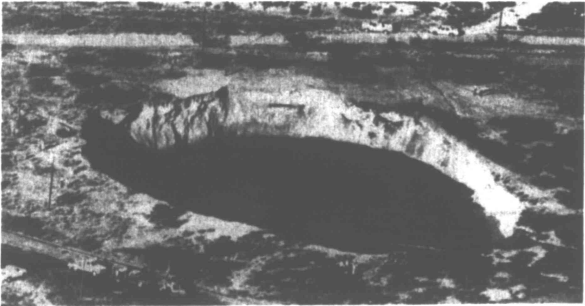
SINK HOLE GROWING — Aerial view from 400 feet shows a growing crater about the size of a football field with the depth from 30-60 feet. It formed yesterday morning (Tuesday) near FM 115 between Kermit and Wink. Indications late Tuesday evening showed surrounding
