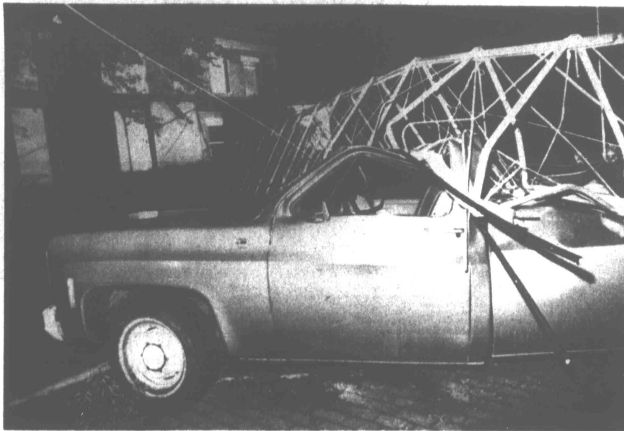
TULIA TORNADO DAMAGE — A large radio antenna, located in Swisher County about 60 miles south of Amarillo, was toppled by a tornado Wednesday night. The twister caused scattered damage throughout the Tulia area. Tulia is located in Swisher County about 60 miles south of Amarillo. There were no injuries reported as of midnight Wednesday. (See related story page 3-A).
