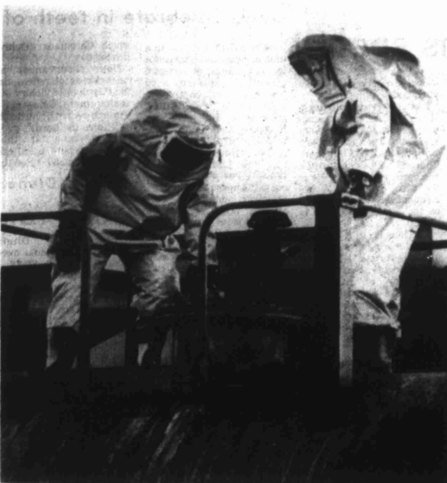
DRAIN TANKER - Workers wearing special protective clothing drain the remaining phosphorous trichloride from a leaking tank car in the railroad yard of Boston & Maine Railroad Thursday night. The rupture in the tanker occurred when a switcher engine rammed the car while it was parked at a siding in the Somerville, Mass. yard. Thousands of people were evacuated from their home as the toxic chemical drifted with the wind.
