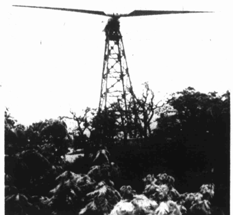
WINDMILL MAY BE WHITE ELEPHANT — This is the world's largest electricity-generating windmill sitting atop Howard's Knob in Boone, North Carolina after it was dedicated July, 1979 at a cost of $3.5 million dollars. The twin-bladed wind machine does not work despite the fact it is one of NASA's pet projects. Many residents in Boone have taken to poking fun at the structure and two residents have made a comedy film about windmill.
