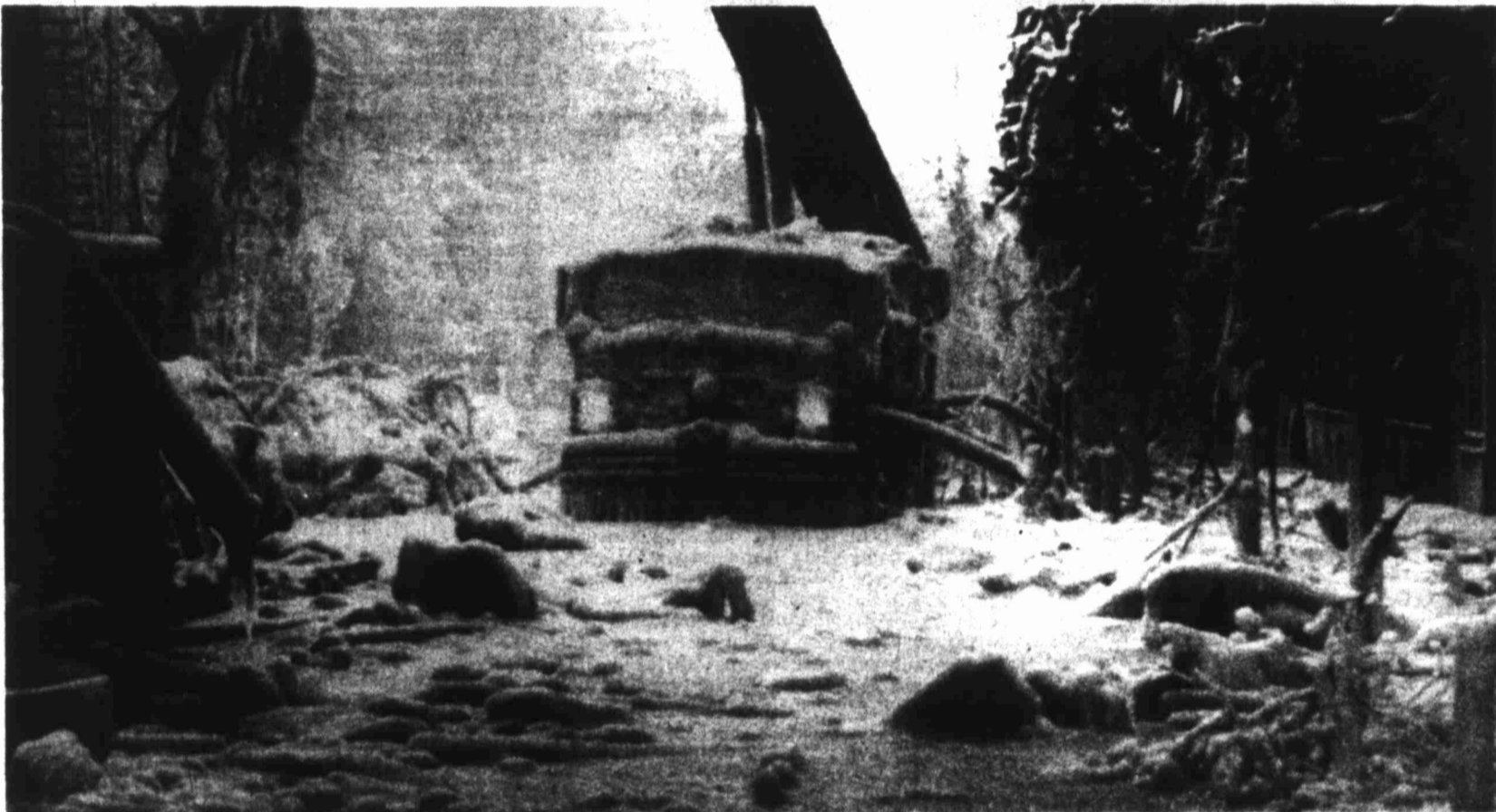
FIRE AND ICE — An ice-encrusted New York fire truck stands in the midst of an eerie cityscape in Brooklyn Heights Friday. The scene is the result of attempts to extinguish a five alarm fire at a ten-story hotel being renovated in
