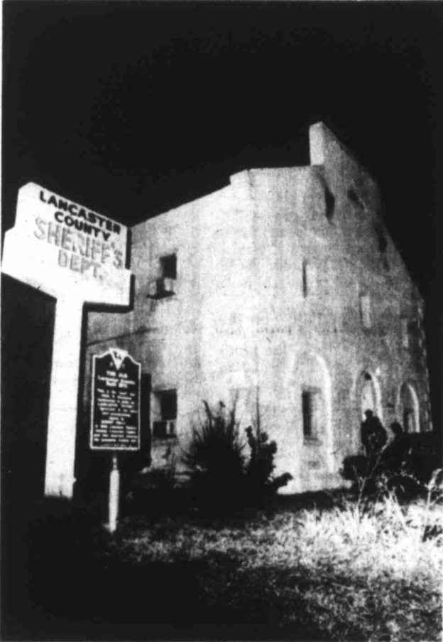
JAIL FIRE KILLS 10 — Ten inmates trapped behind bars died when a fire broke out about 6 p.m. Thursday on the second floor of the Lancaster County jail in South Carolina. The inmates died, apparently after breathing smoke from burning mattresses.
