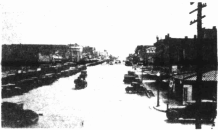
Looking South on Main St. in 1928 the original stores that were to become the now familiar Big Spring Hardware and Furniture.
