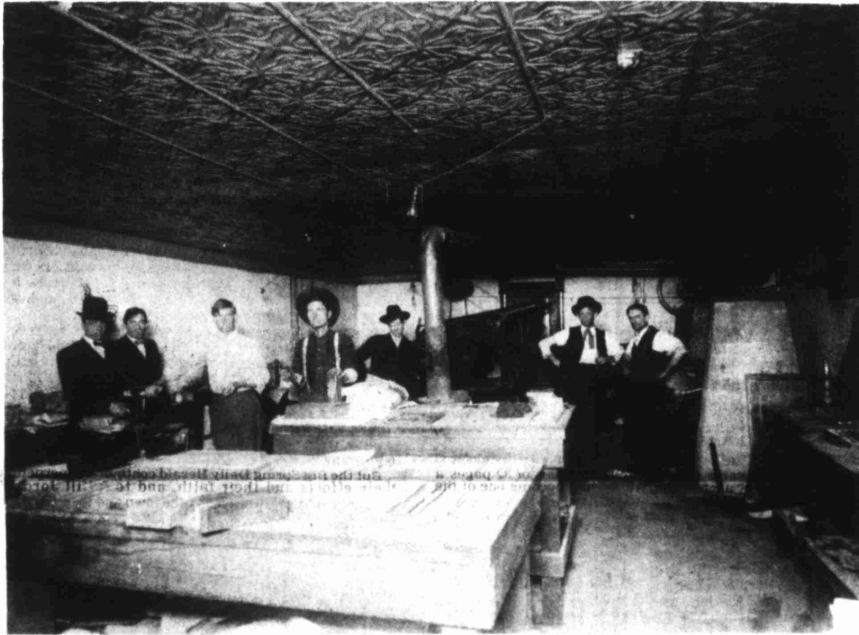
PRINTING METHODS RATHER PRIMITIVE — Five years after it was founded, the composing room of the Big Spring Herald looked this way. The scene was set in 1909 in the basement of the old Ward Building at Second and Main Streets. Pages were assembled on stone-topped tables and printed on a flat-bed press. W.G.
