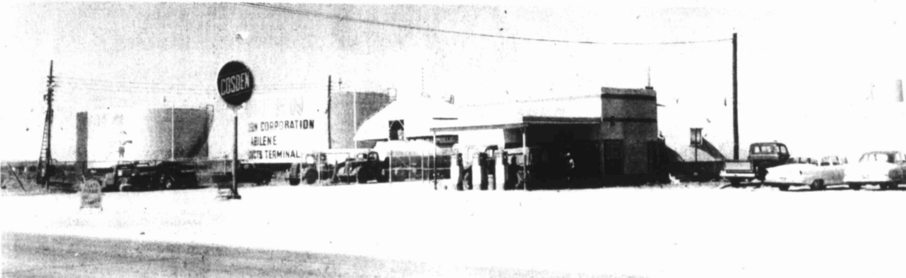
SUBSTATION OPERATION — Cosden Oil and Chemical Co., maintained a terminal in Abilene for many years. At one time, Cosden also maintained a service station beside the terminal. That occurred in the 1950s, before Cosden ceased to manufacture
