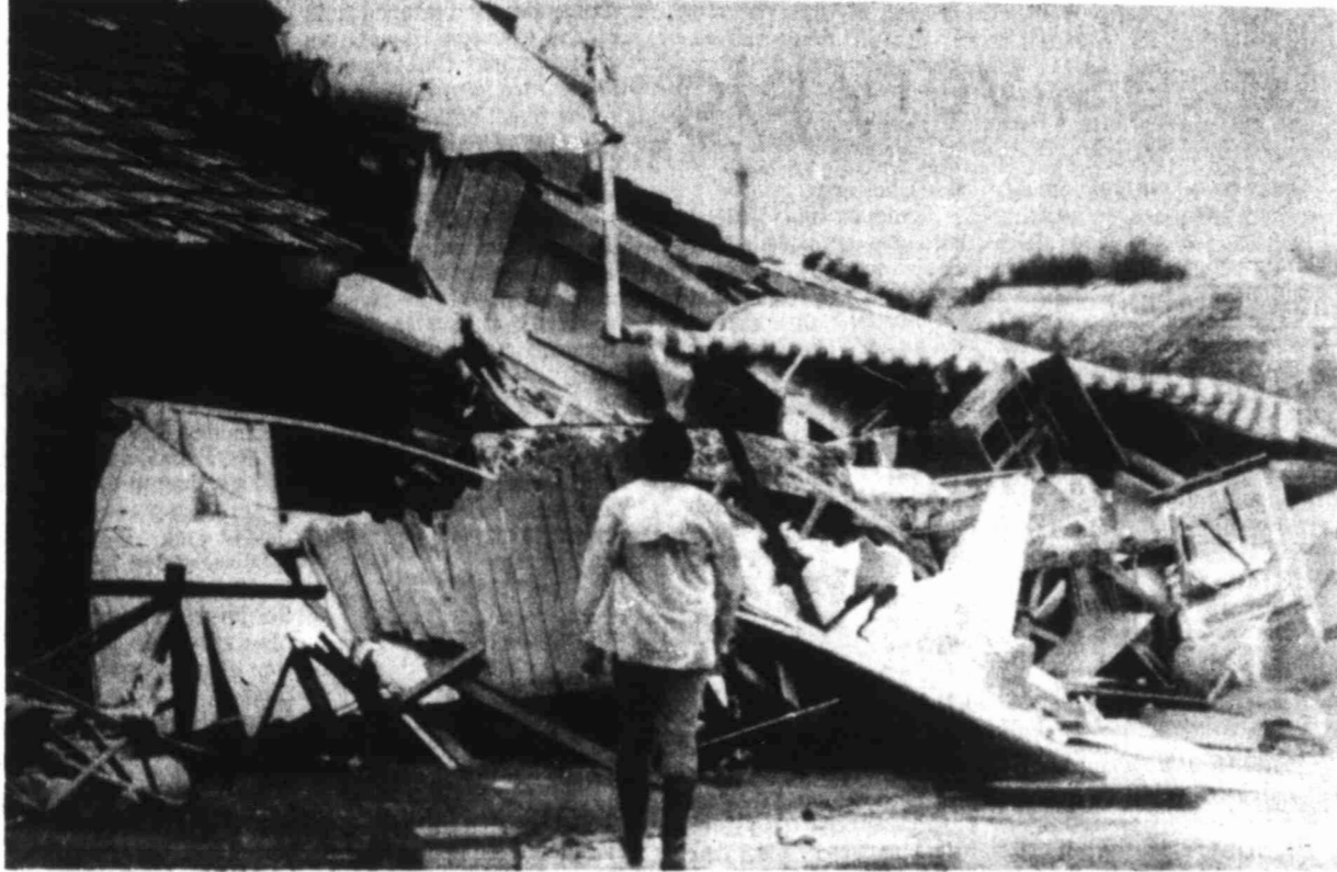
WIND SWEEP TRAILER — A House trailer rests against the side of a building after being thrown across a street at the Ocean Holiday Mobile Home park in Melbourne Beach. Several mobile homes were destroyed due to winds from Hurricane David.
