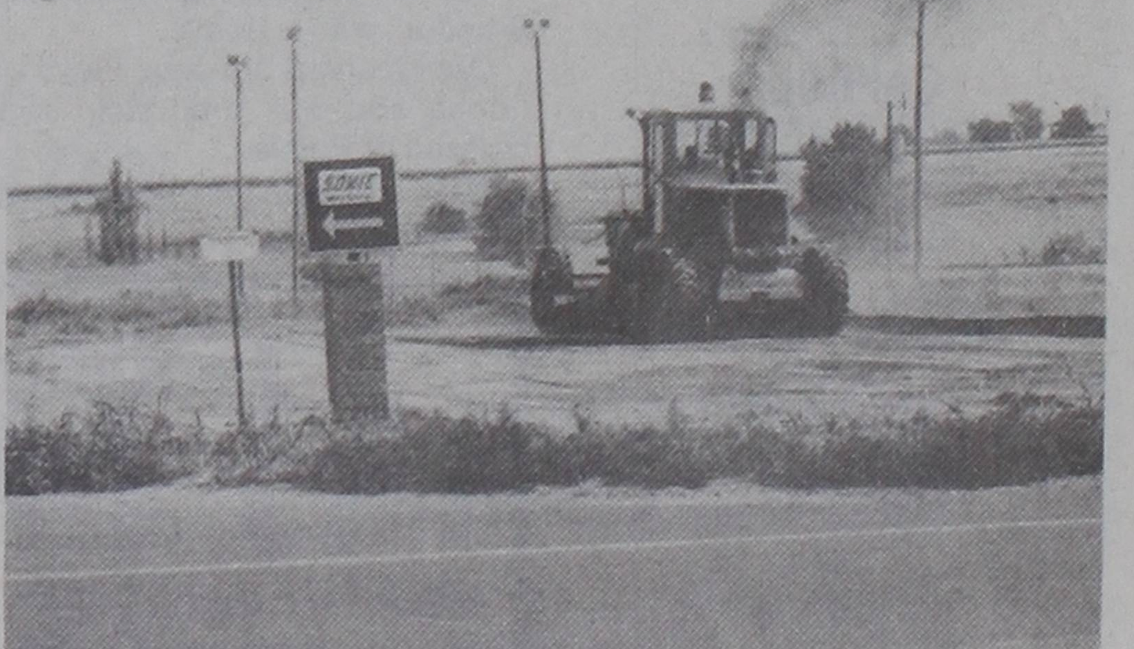
DIRT WORK....A motor grader is shown doing dirt work for part of the Lakeside Addition project, which got underway this week. First homes in the project are expected to be completed by the end of September.
