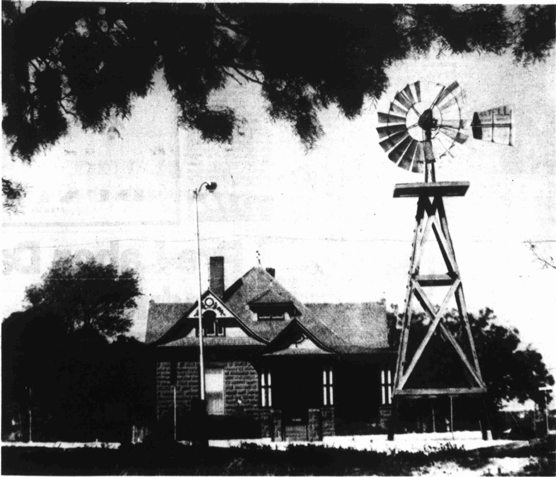
STORIED RESIDENCE — The Potton House, located at Second and Gregg Streets, has become one of Big Spring's most famous landmarks. The house has been restored with the help of public funds and private donations and is open for tours. The windmill pictured in front of the house here is, in reality, across the street and, of course, is not visible. Here, photographer Danny Valdes catches the magnificence of the Victorian house, which has been in existence for 78 years.
