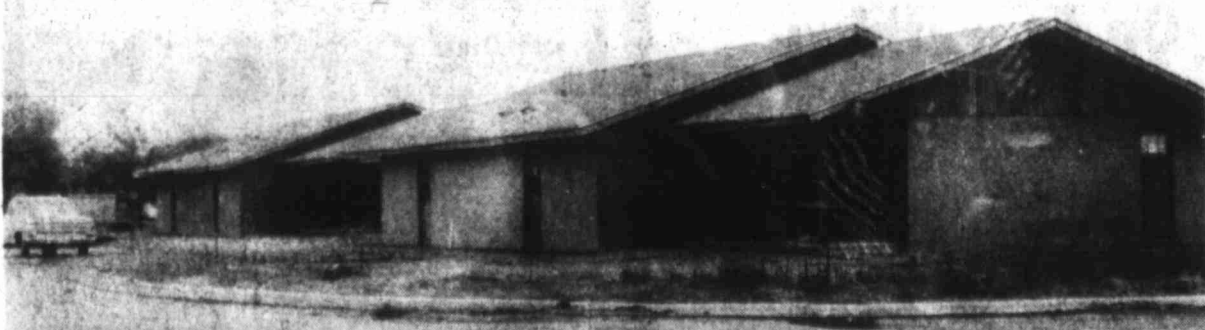
NEW HOME — Four new cottages will soon house the Work Village at Big Spring State Hospital. Each cottage will hold eight residents. Cooking facilities are included
