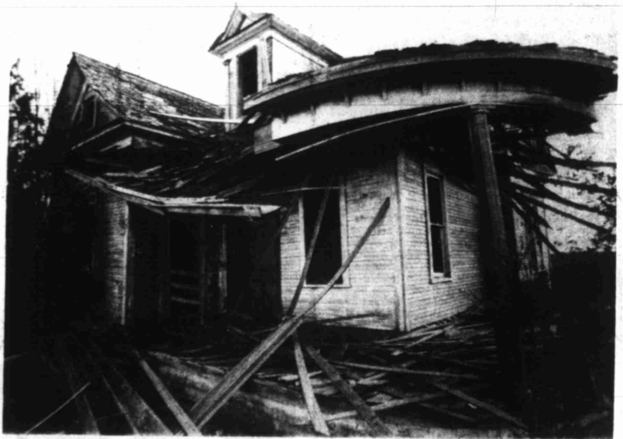
CURVED-PLANK PORCH AND GABLED, WOOD-SHINGLED ROOF SHOW SIGNS OF PAST GRANDEUR ... built in 1904 by carpenter named Rogers who did work on county courthouse
