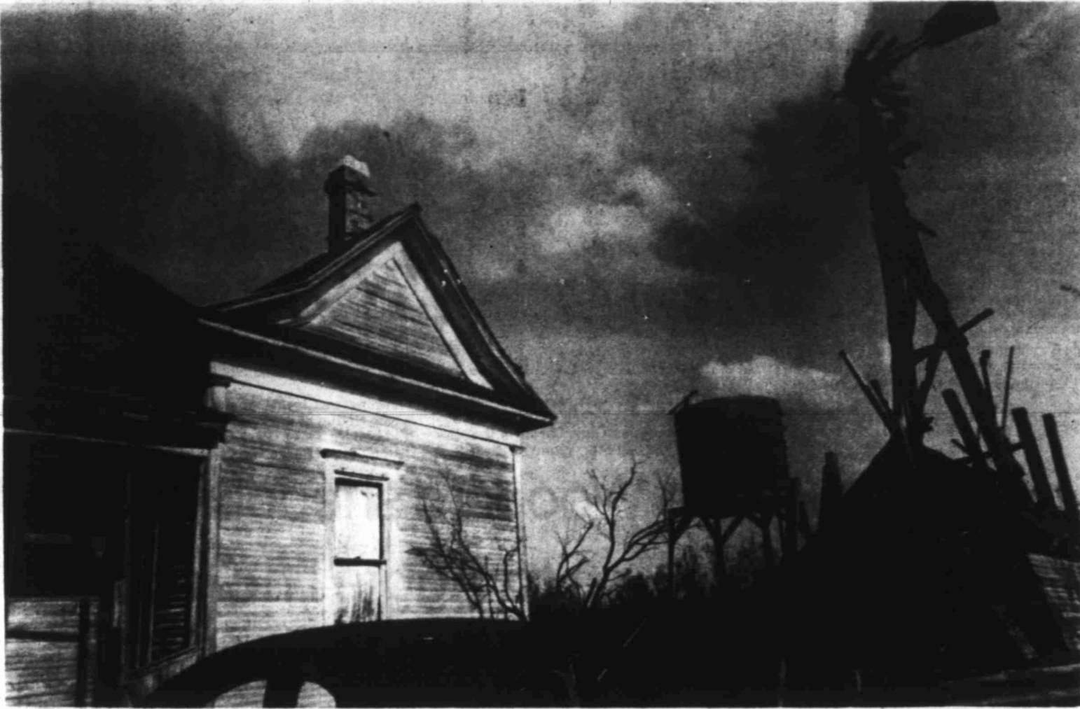
WEST TEXAS WINDS WREAK DAMAGE ON THE WINDMILL AND HOME ... and located just west of Garden City on Texas Highway 158
