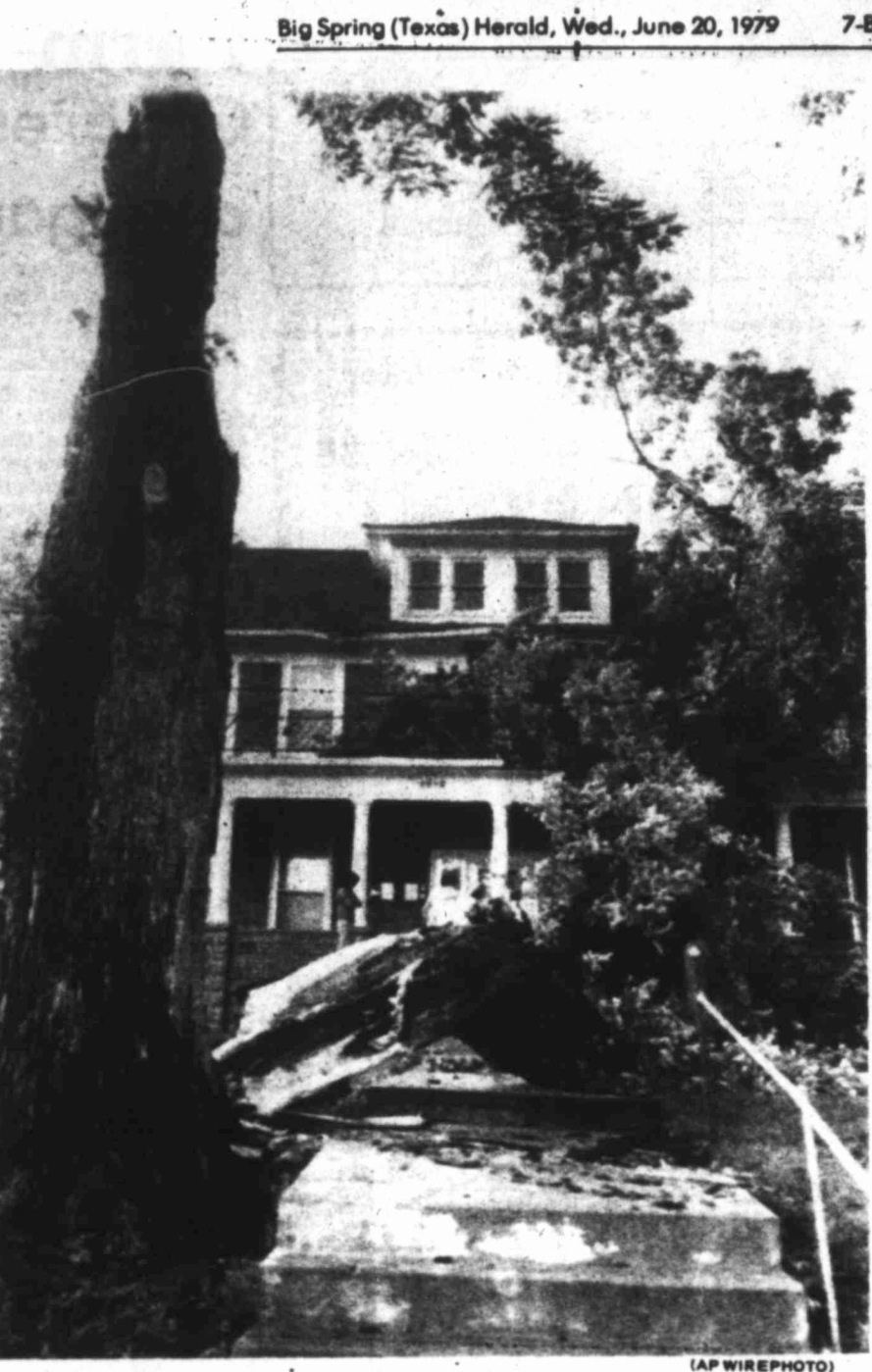
MAPLE FALLS - A 50-year-old, 100-foot high male tree is toppled by high winds that hit midtown Omaha Tuesday. The tree damaged the roof and porch of an apartment building owned by Ron Fehr. Tornadoes, funnel clouds and severe thunderstorms swept over much of eastern Nebraska in the late afternoon and early evening.
