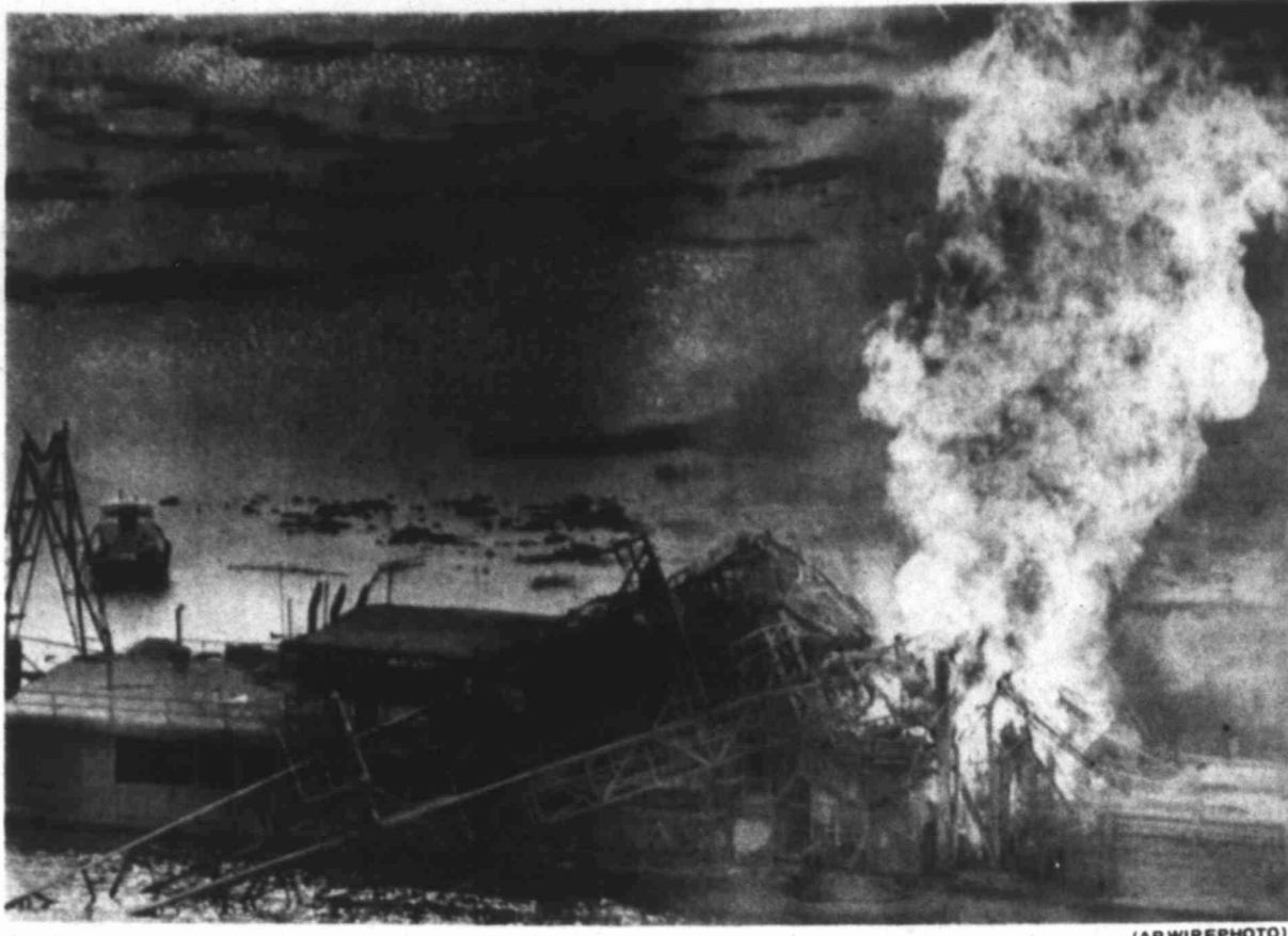
FIERY GAS RIGGING — Flames shoot from a drilling rig in marshes about 50 miles south of New Orleans, La., where natural gas exploded and caught fire Tuesday, severely burning four crewmen. At the time, workers were pulling up a drill on the Texaco rig.
