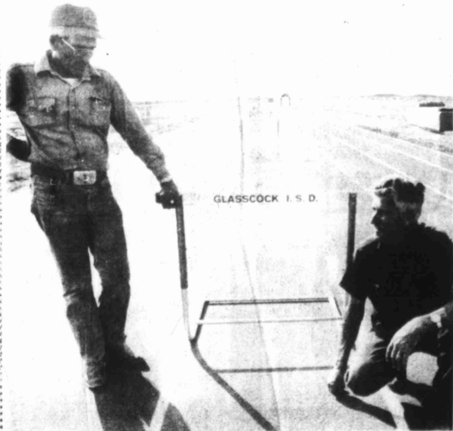
ONE OF TWO IN STATE — W.J. Livingston (left), a member of the Glasscock County school board, is shown conferring with George Smith, who is helping put the finishing touches on a new $100,000 track at Garden City High School. The track, which provides a suitable cushion for runners, is one of two such tracks in the state. The other has been built at Wichita Falls. The surface is 80 per cent rubber and 20 per cent asphalt.
