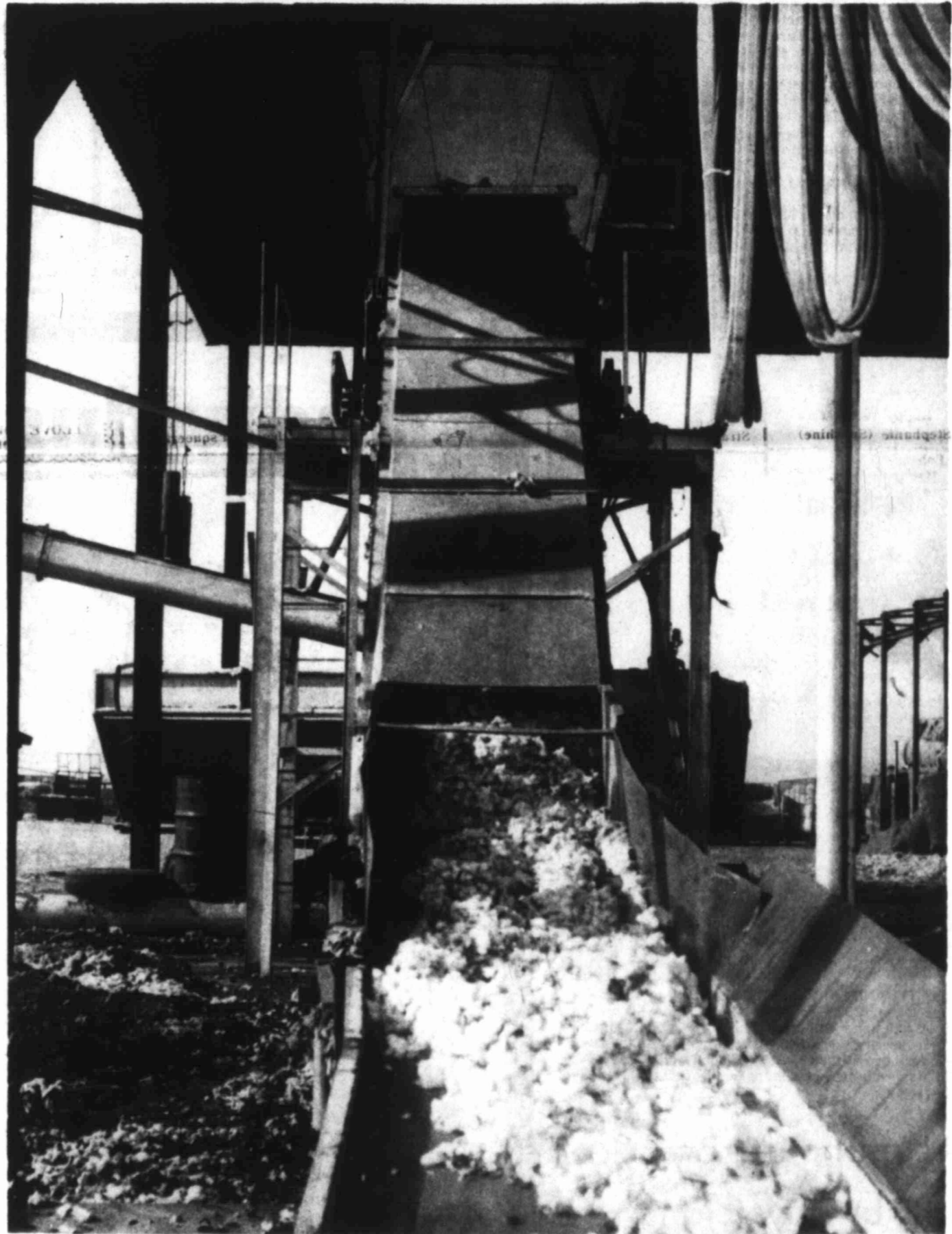
... on metal pathway to machinery inside ...
