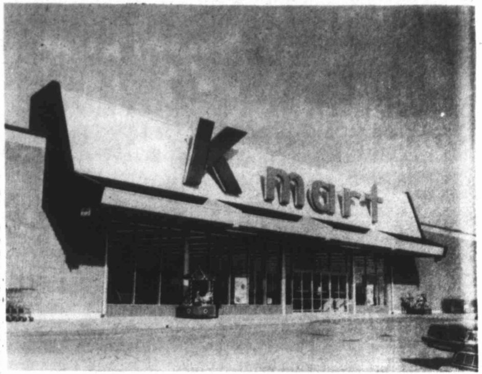
THRIVING CONCERN — The long awaited Kmart store, opened during the fall of 1978, decorates what promises to be a major shopping area in the southeast section of Big Spring. It is located just off Birdwell Lane and FM 700.
