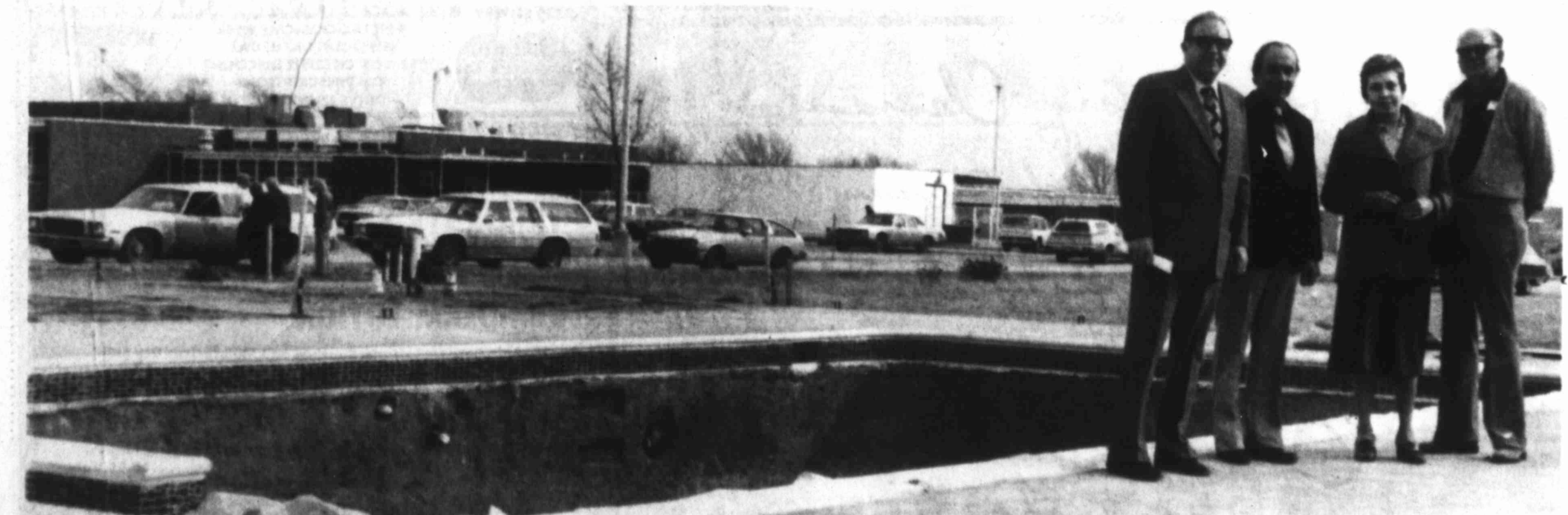
REALITY — In 1976, the Volunteer Services Council of the Big Spring State Hospital began its fund-raising campaigns for a therapeutic swimming pool for BSSH patients. Completion of the pool is estimated to be around the middle of March. Pictured here, left to right, are A. L. Gatewood, director of rehabilitation services at BSSH; Ned Abraham, representative of Levi Strauss Company of Midland; Grace Ferguson, M.D., M.P.H., BSSH superintendent; and Jack Y. Smith, chairman of the swimming pool project and treasurer of the Volunteer Services Council.
