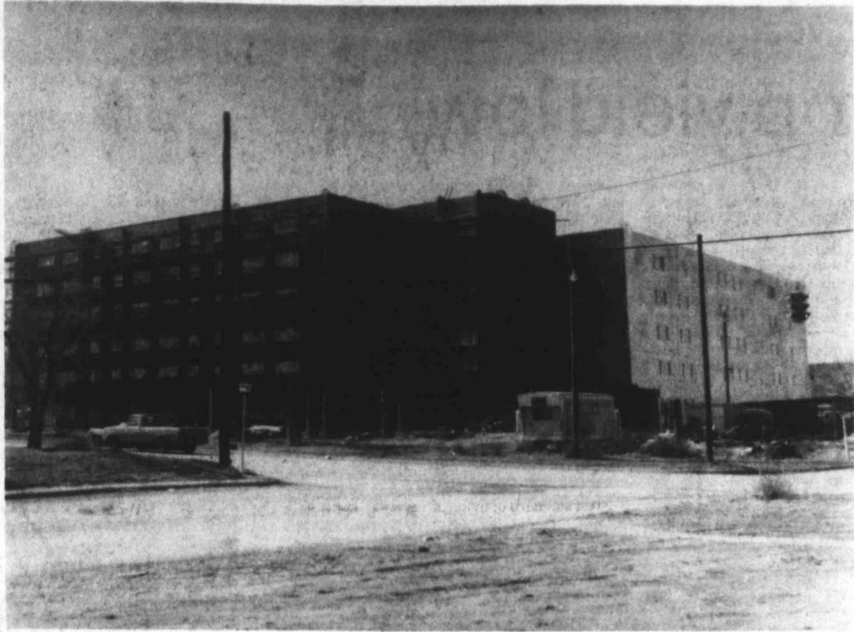
SCHEDULED TO OPEN THIS YEAR — The opening of the Canterbury Retirement Center, located at 17th and Lancaster Streets, is scheduled this year. The handsome structure is being built by a board composed of members of St. Mary's Episcopal Church, who obtained a
