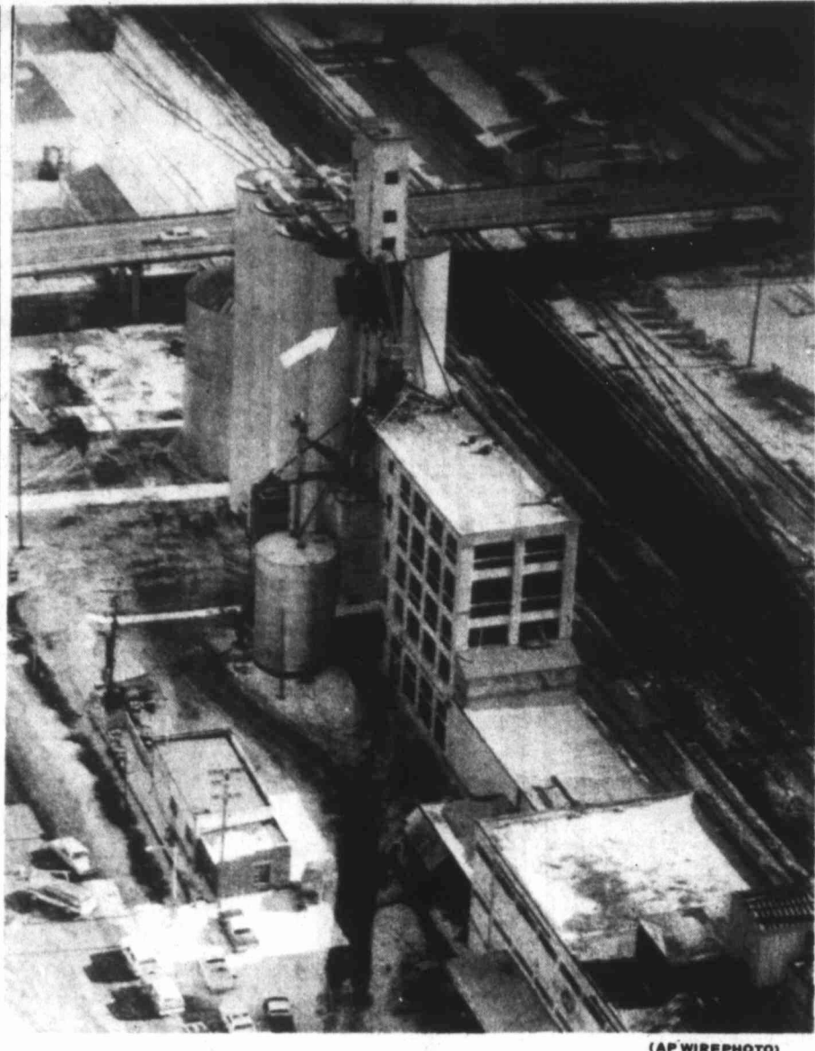
ELEVATOR EXPLOSION — An aerial view shows a hole in the grain elevator at Lexington, Neb., after an explosion ripped through the building Tuesday. One man was killed and another remains in critical condition. The blast threw the men approximately 120 feet to the ground. The blast did not cause a fire.
