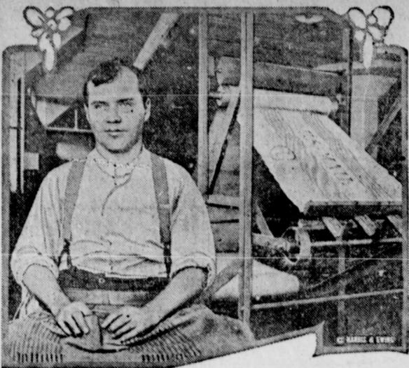
With a capacity of eight bags a minute, this machine, recently built and installed in the mail shops of the United States post office department, displaces the services of eight men, cutting, stenciling, folding and stitching the canvas cloth at a single operation. William Allen West, shown in the illustration, who has been putting the cords through mail bags in the equipment shops since 1917, has been blind for 20 years. He has a capacity of 325 bags a day.
