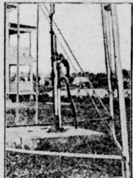
Tightly Fastened Pump and Curb.
