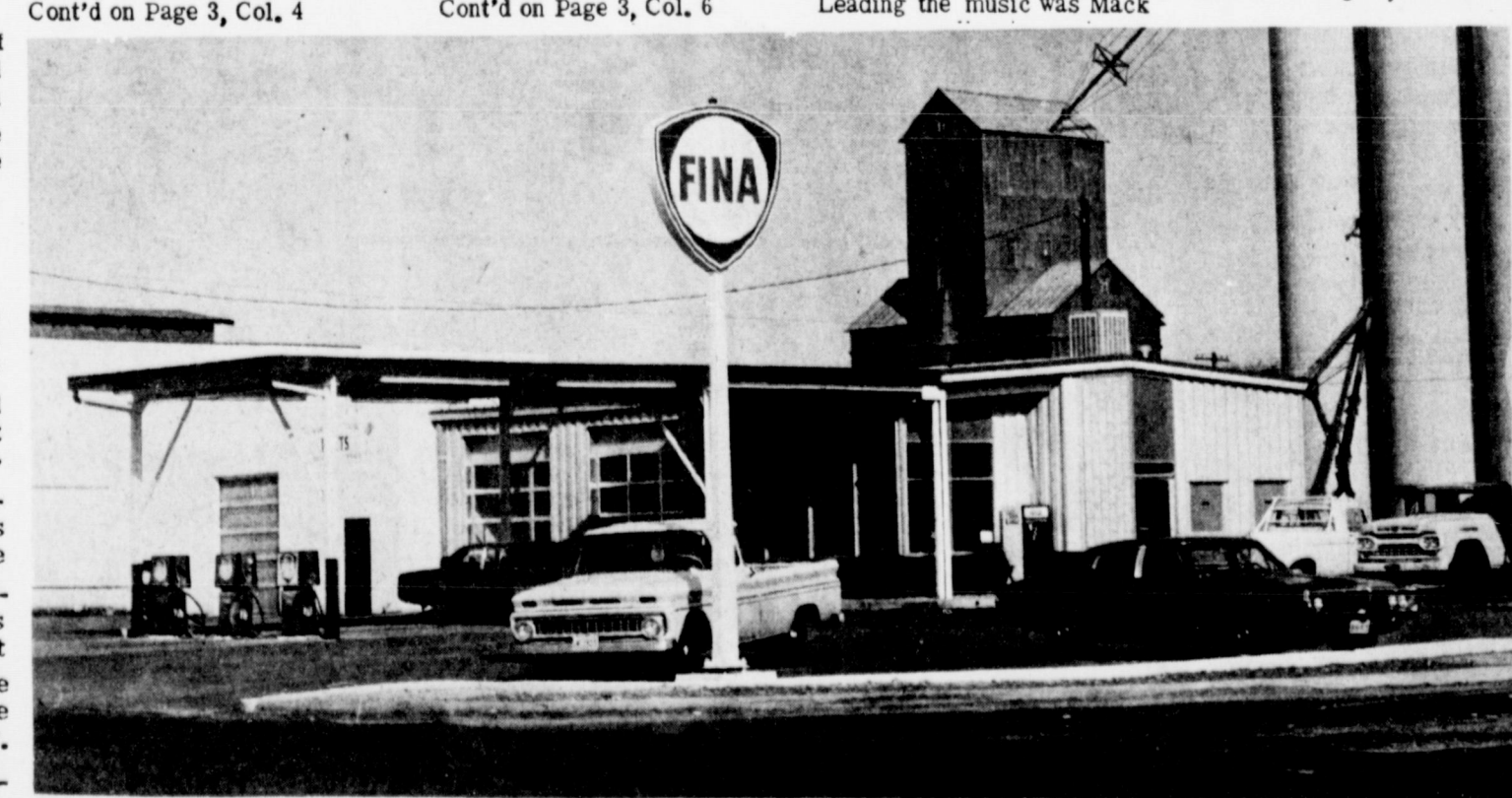
VIEW OF NEW HOLT'S FINA SERVICE STATION--Recently completed is the all-new Holt's Fina Service Station at the intersection of Highways 84-70 in Muleshoe. Grand opening for the new station will be Saturday, December 6. Prizes and gifts will be awarded throughout the day. Operators of the station and wholesale business are Mr. and Mrs. Clyde Holt. A Holt service station has been in operation continuously at the same location since 1932.
