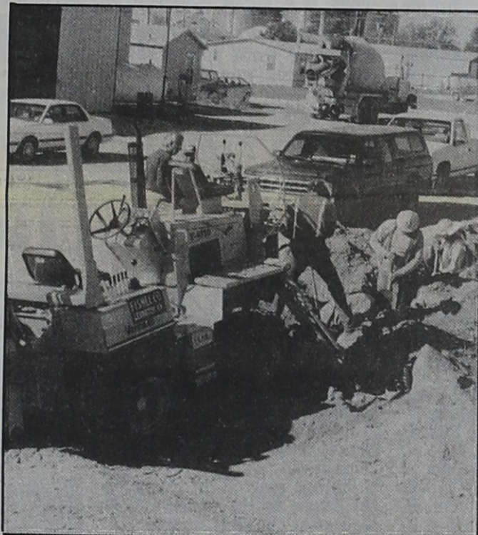
Our Line-laying Crew
