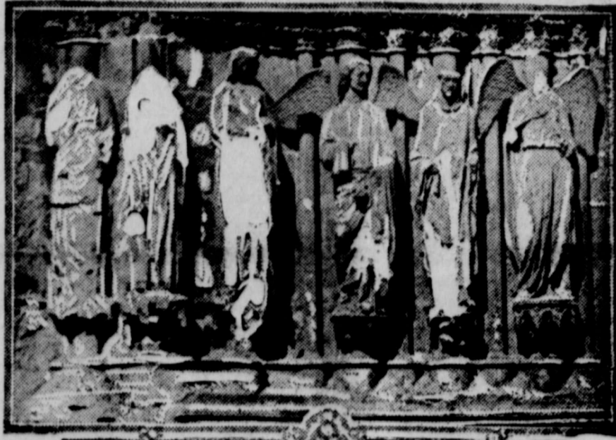
1914, by American Press Association. This shows merely a small section of the outer wall on which the damage done to the statues by the German shells is plainly seen.
