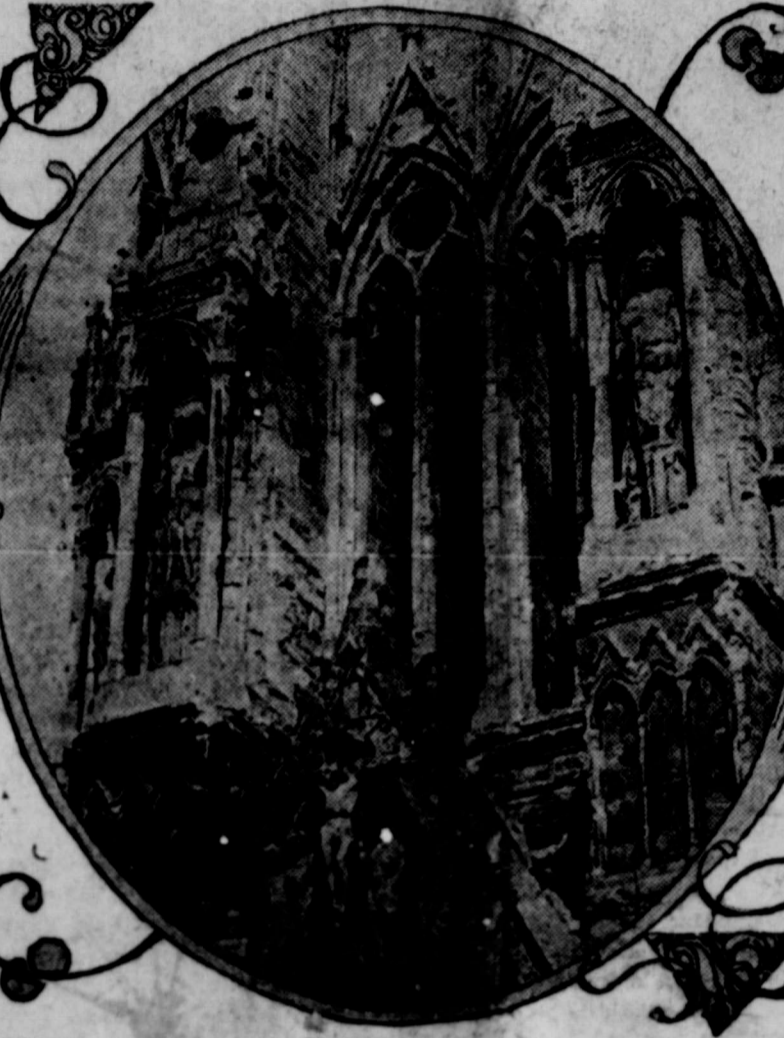
© 1914, by American Press Association. View of one wall of the edifice after the bombardment.
