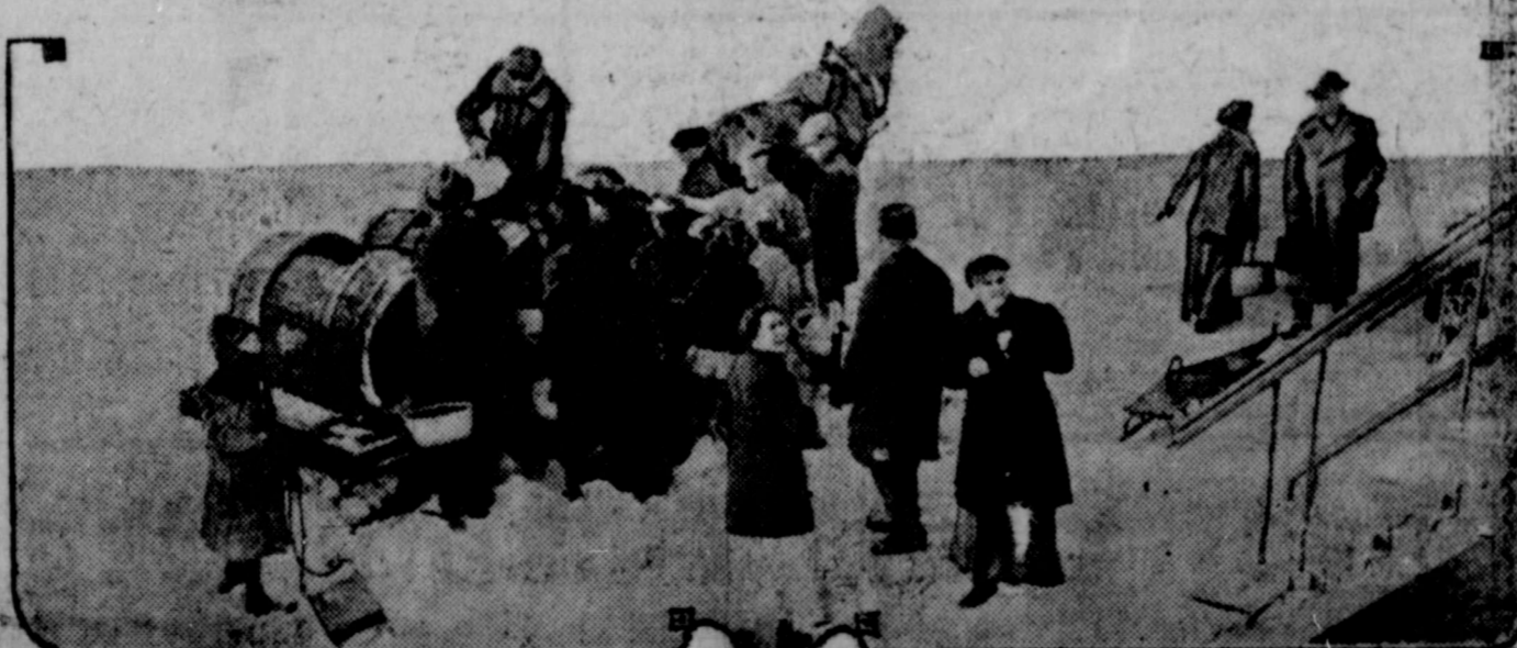
Montreal has been struggling with a serious water famine caused by the breaking of a big conduit, and the result was a great conflagration. Wagons carrying water went up and down the streets occasionally, announcing their coming by the ringing of bells, and supplying the residents with water for their household needs.
