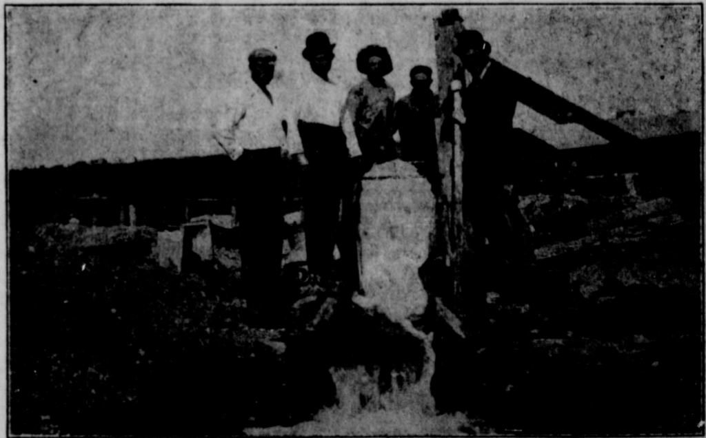
THE ALLEY WELL, HALF MILE FROM HALE CENTER—1,500 GALLONS A MINUTE.
