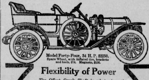
The Offset Crank Shaft is what gives the Rambler engine its flexibility of power. The Rambler will run smoothly and quietly on high gear at 3 or 40 miles an hour. It allows the owner to conform easily to the limitation of the traffic without conform to the conformation. tions of congested city traffic, without constant gear changing.
