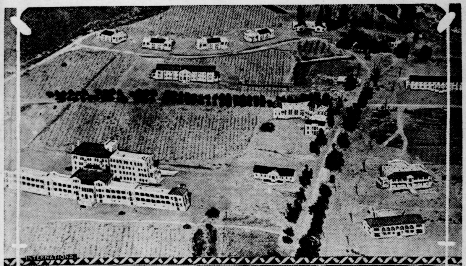
Airplane view of the buildings and grounds of the United States government hospital under construction at San Fernando, Cal. The structure in the right middle foreground was wrecked recently by an explosion.
