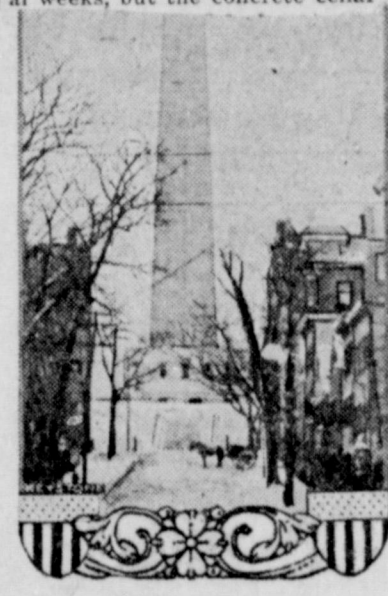
New view of Bunker hill monument, looking up Monument street from Medford street, Charlestown, Mass.
