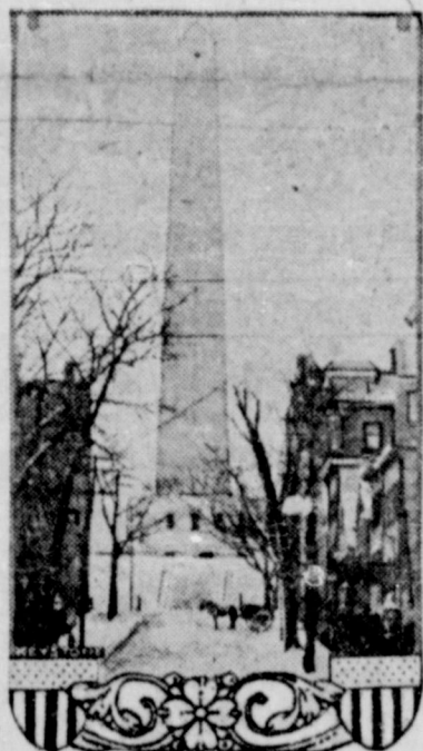
New view of Bunker hill monument, looking up Monument street from Medford street, Charlestown, Mass.
