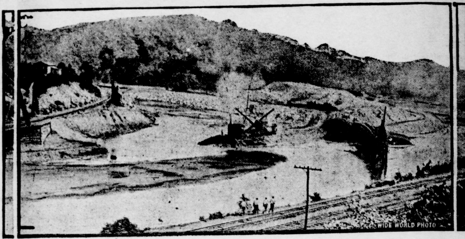
The setting off of 1,700 pounds of dynamite completed the great engineering project of moving the Schuylkill river a distance of a half a mile at Port Clinton, Pa. The new road for which the course of the river was shifted represents an expenditure of $500,000 and eliminates a "U" curve and two obsolete bridges. Photo shows the new channel of the river at the left and the old one at the right.
