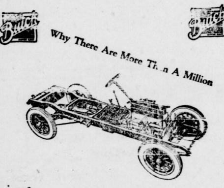
The Buick "Sealed Chassis"! From front to rear, a continuous wall of iron and steel housings behind which the Buick driving units operate. Dirt and wear kept out-lubrication kept inl Only Buick has all of this protectic a. Another big reason why the Buick name is a synonym for reliabilityand why there are more than a million Enick owners.
