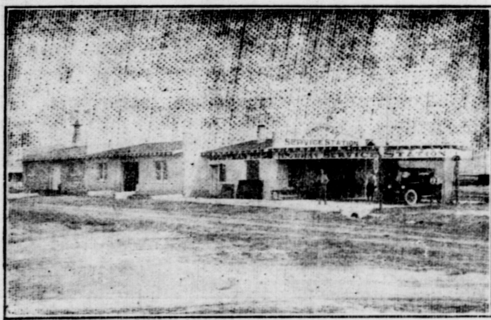
HIGHWAY SERVICE STATION
