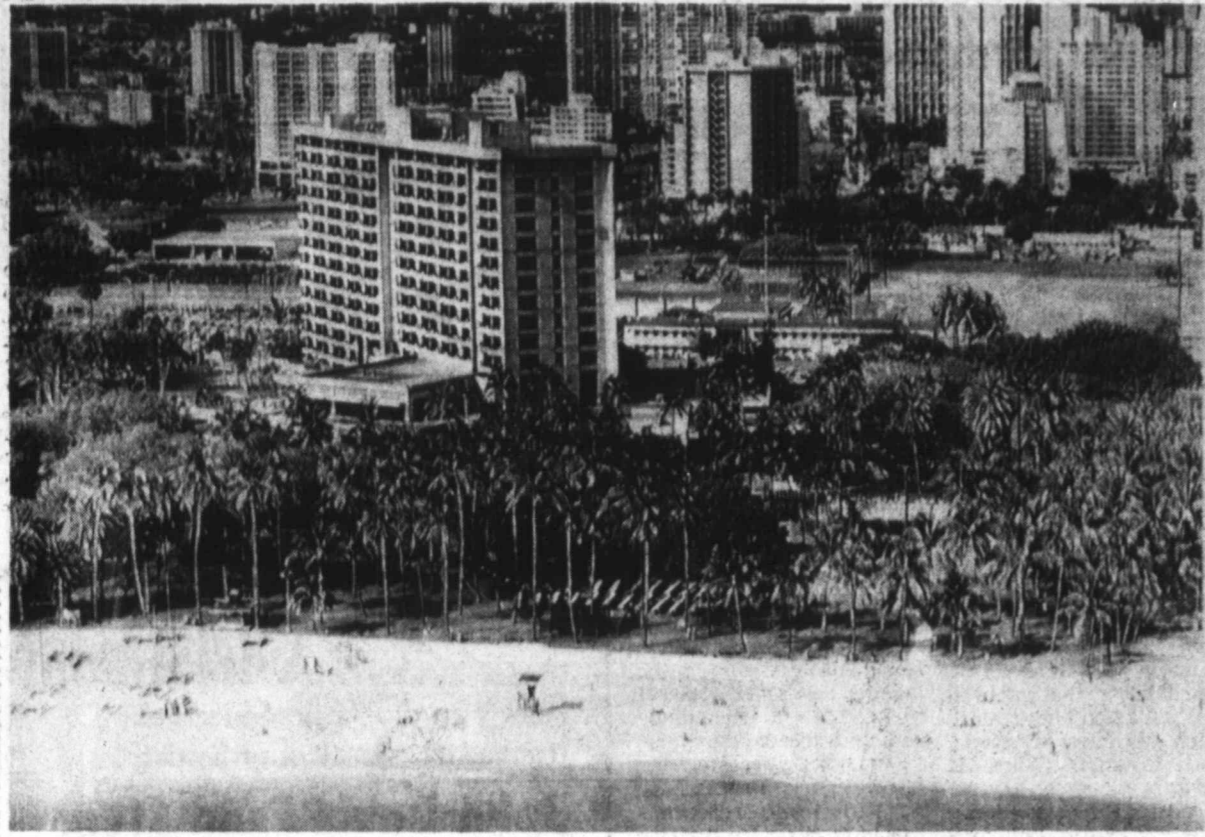
MILITARY HOTEL — The government-run Hale Koa Hotel on Hawaii's Waikiki Beach, center foreground, is getting about $1 million a year from taxpayers and is being used chiefly by retired military personnel, ac-
