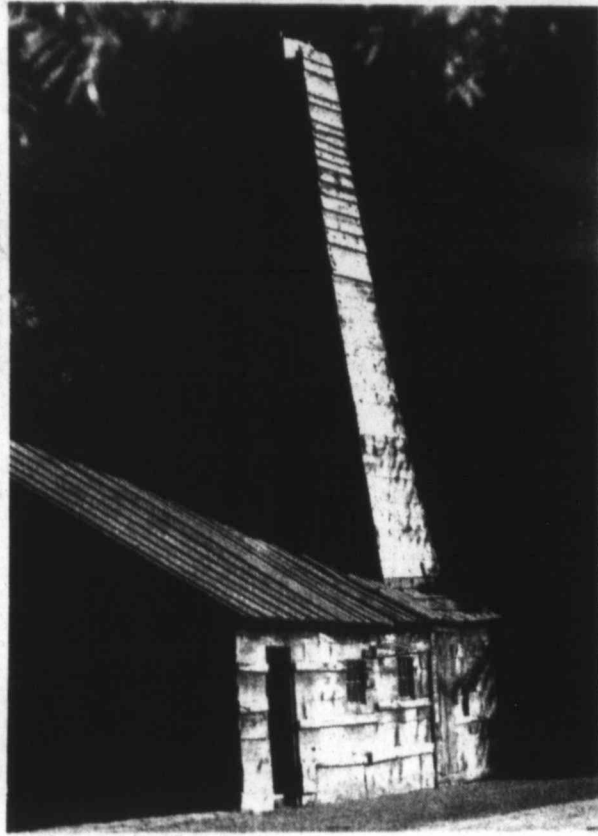
SECOND WELL — Drake Number Two, America's second oil well, has been restored at the Drake Museum in Titusville, Pa.
