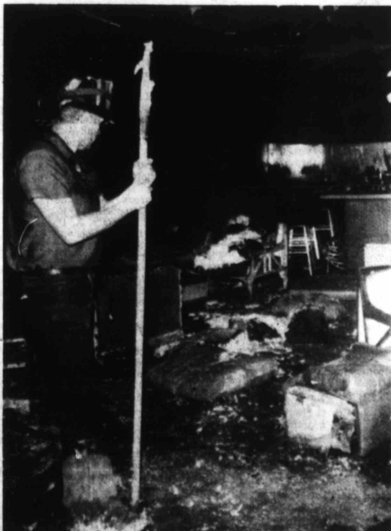
SURVEYS DAMAGE — A New York City fireman surveys damage to the Sir Harry's Bar just off the lobby of the Waldorf Astoria Hotel in New York Sunday night. Witnesses said a man police identified as Cary Jon Yurman, 32, of San Francisco, left the bar after a dispute, then returned and threw a lit can of gasoline into the bar. Yurman was arrested and charged with arson after allegedly setting the fire.
