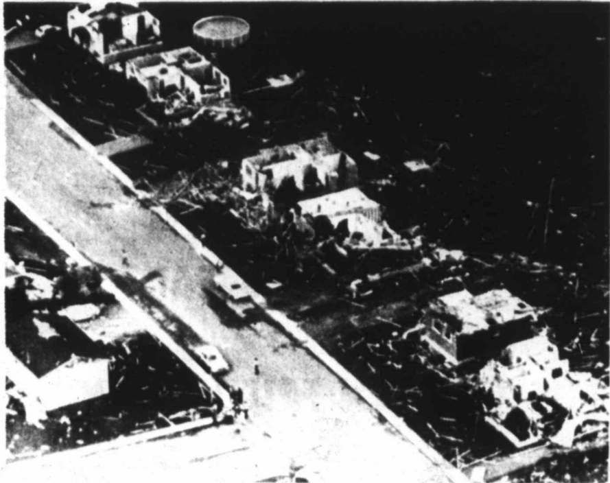
TORNADO'S TRAIL — These are some of the 65 homes that were smashed Tuesday by a tornado that swept through Buckingham, Quebec. About 34 persons were injured in the two-minute storm.
