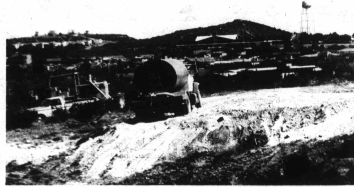
STREET PAVING, UTILITY INSTALLATION AND LOT PREPARATION ACTIVITY
