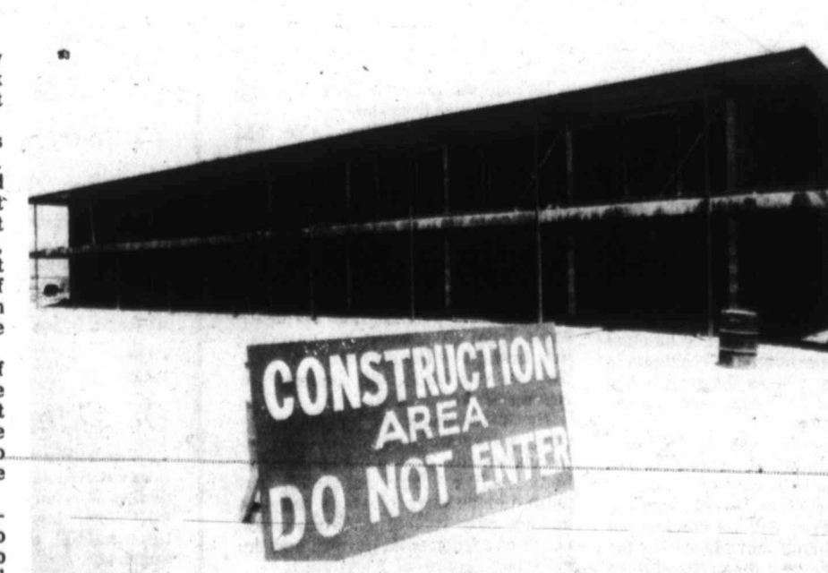
GOING UP — An addition of 32 rooms at Mid Continent Inn will make room for more customers for the one-year-old motel which is usually full and running over.
